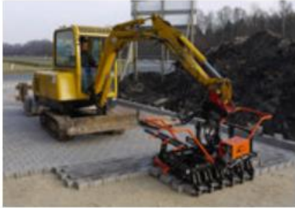
Paving by excavator with the Optimas clamp.
