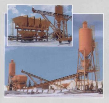
This plant requires easily replaceable aggregate bins because it is located in the Bahamas and the aggregate is washed with highly corrosive salt water. These bins supply material to an open air Findlay block machine as well as a ready mix fleet. It is swend by faland Construction Co.
